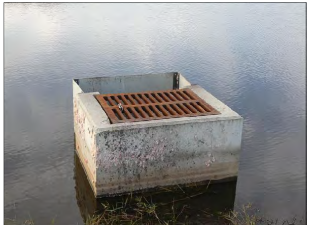
Stormwater Drainage Control Structure
