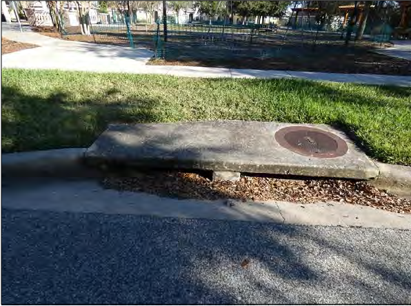
Stormwater Drainage Curb Inlet
