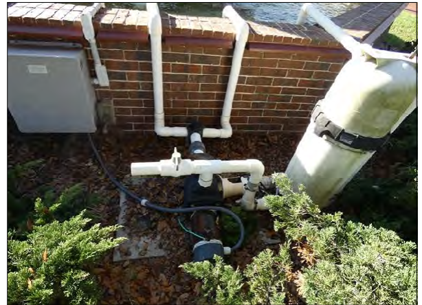
Connerton Blvd Fountain Equipment, Note Rusting Pump
