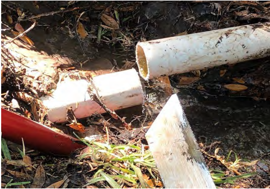
The tree root growing between the two zone pipes in zone A50 bowed the pipe by over an inch.
